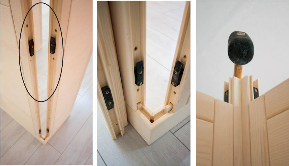
Fig. 4: Connecting wall elements with corner post
