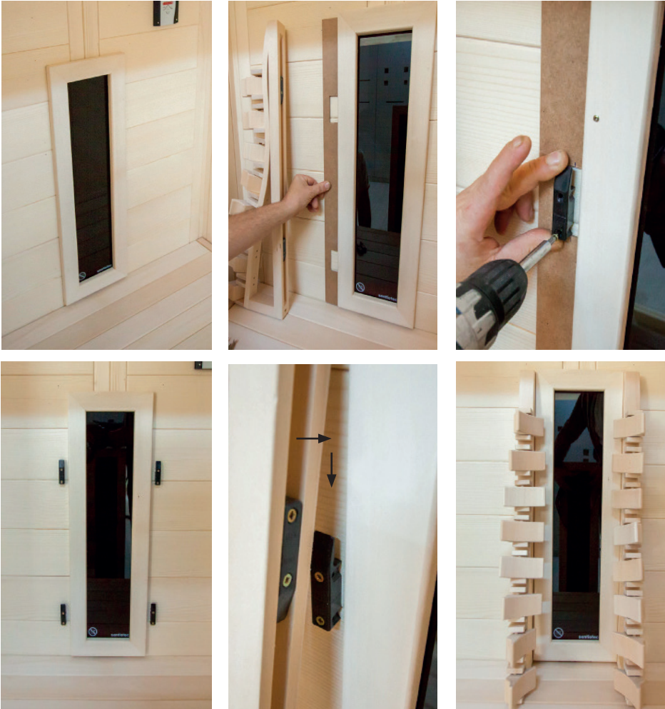
Fig. 29: Installing the backrests
