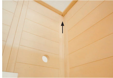
Position of slat with drill hole
