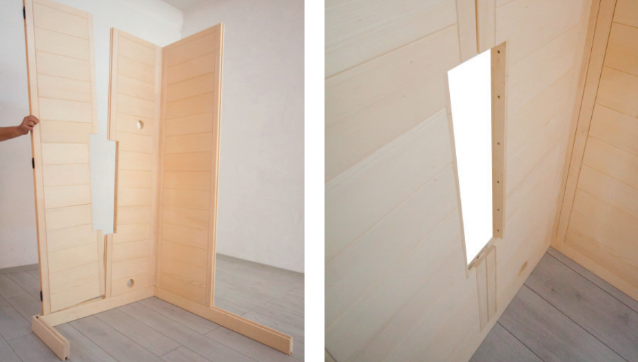
Fig. 6: Inserting wall element with recess
