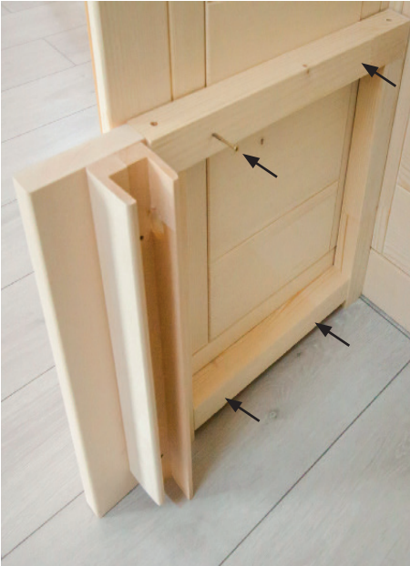
Fig. 18: Installing the bench supports
